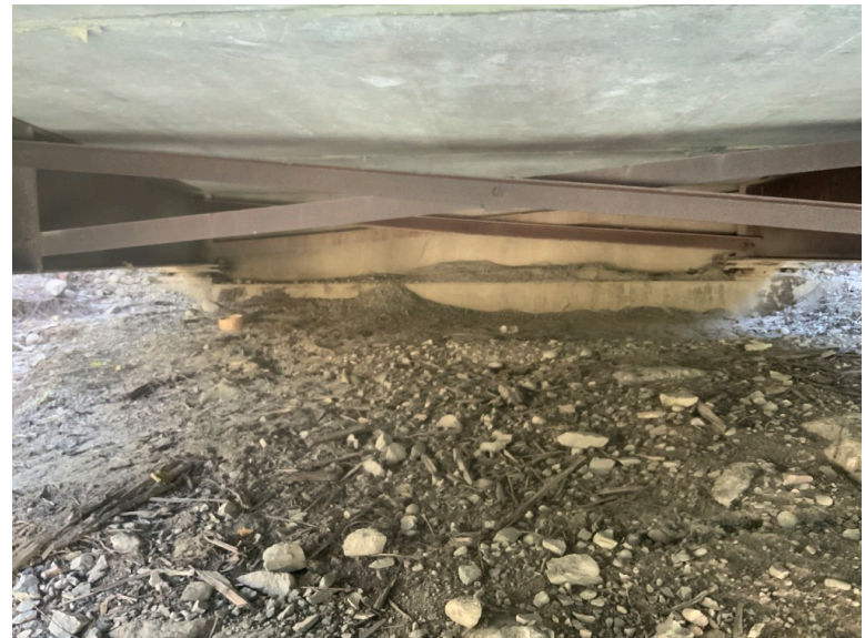
Left Bank Abutment when facing downstream
