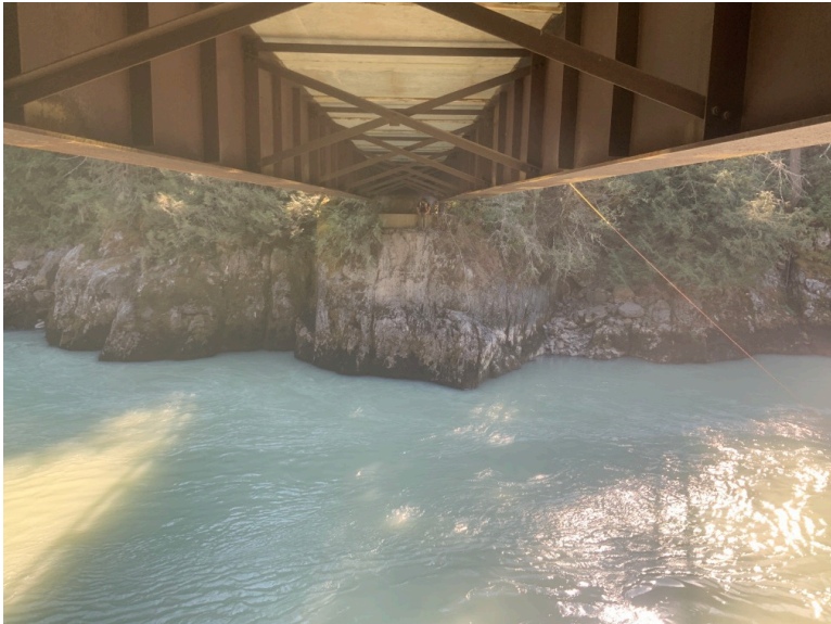
Left Bank Abutment when facing downstream
