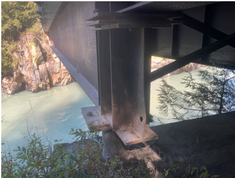
Jump span bearing. Ds. Deformation
