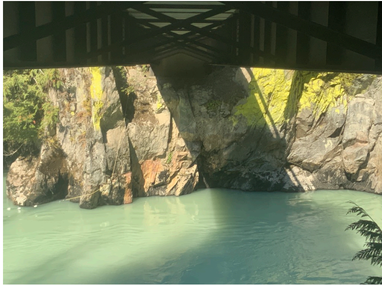
Right Bank Abutment when facing downstream
